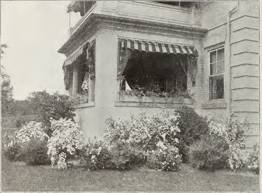
See how much more attractive and valuable a home can be made by a simple planting of shrubbery
