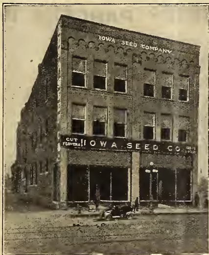
Retail Store and Office Building
