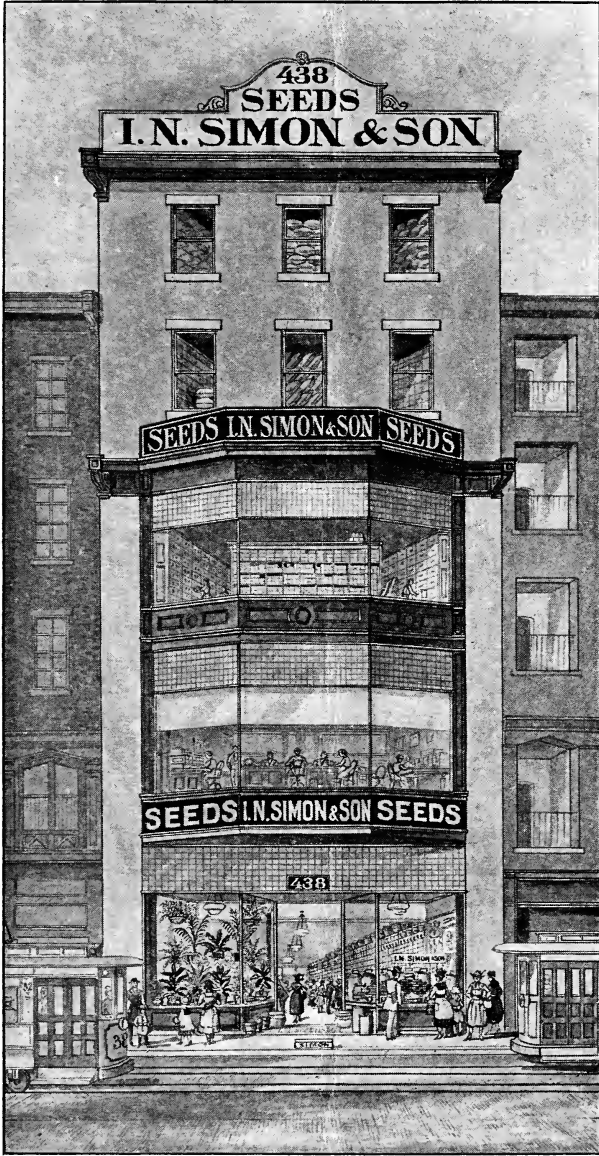
The Above is a Photograph of Our New Store at No. 438 Market Street where we have every Modern Convenience for the execution of orders. It consists of five stories and basement, and runs through to Ludlow Street opposite the Bourse Building.
