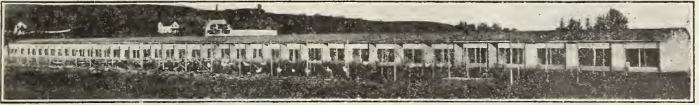
The above is a picture of our new poultry house on our poultry farm adjoining Blair. It is 400 feet long, 20 feet wide, is electric lighted, has three hydrants, root cellar, store room for feed and loft for straw and is probably one of the most up-to-date big poultry houses in America.
