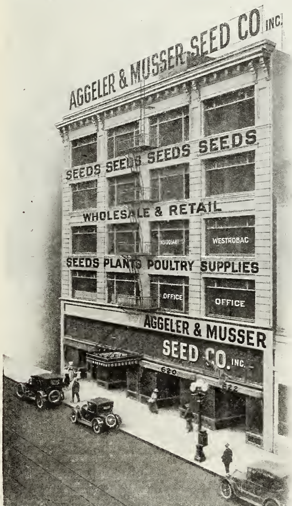
This building is located just South of Sixth, on Spring Streets, One block from the Huntington Building. Convenient to the rural population who daily pass to and from the Pacific Electric Depot.
