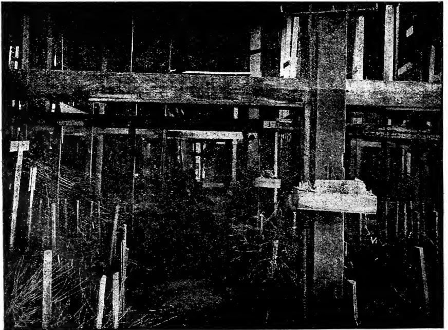
INTERIOR VIEW OF FROST PROOF CELLARS, WHERE STOCK IS STORED FREE FROM ATMOSPHERIC INFLUENCES, DURING PACKING SEASON.
