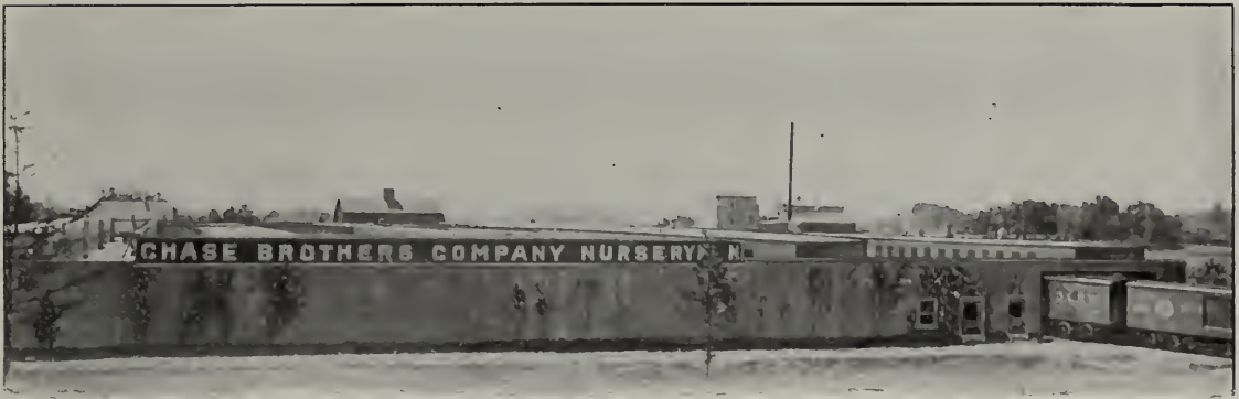
Our Packing Cellars are thoroughly modern and built for the purpose
