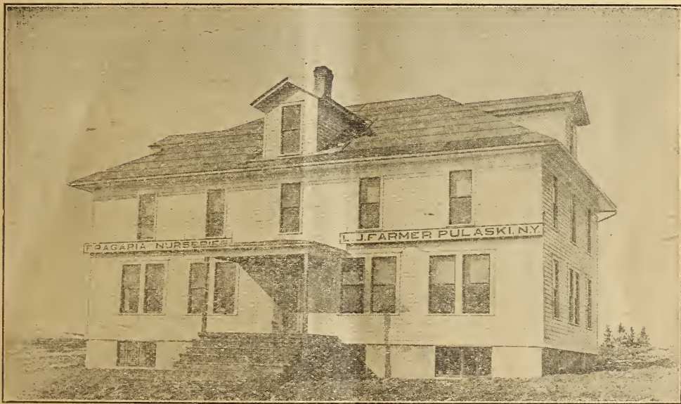
The above picture shows our Office Building occupying a ground space of 30 by 52 feet
