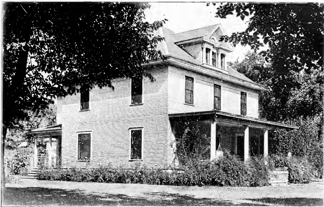
A York home showing the pleasing effect of proper banking of shrubs near the foundation.
