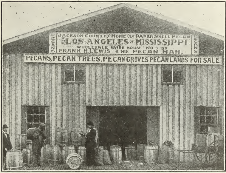
Lewis Pecan Co., Inc., Central Warehouse at Pascagoula, Mississippi.
