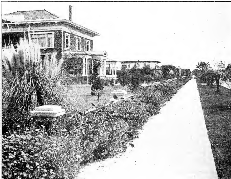
STREET SCENE, MID-WINTER, PHOENIX, ARIZONA.
