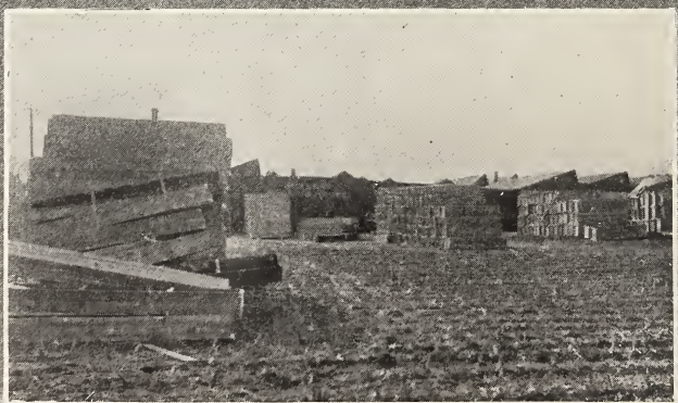
A CORNER OF OUR FROST PROOF PACKING CELLAR
