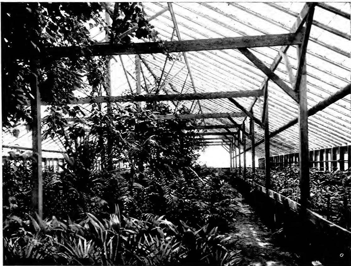
View in One of Our Large Greenhouses
