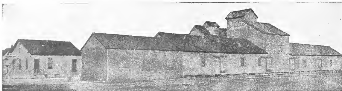
The Disco Offices and Warehouse. Our Corn Drying Cribs are Located Immediately Behind This Building
