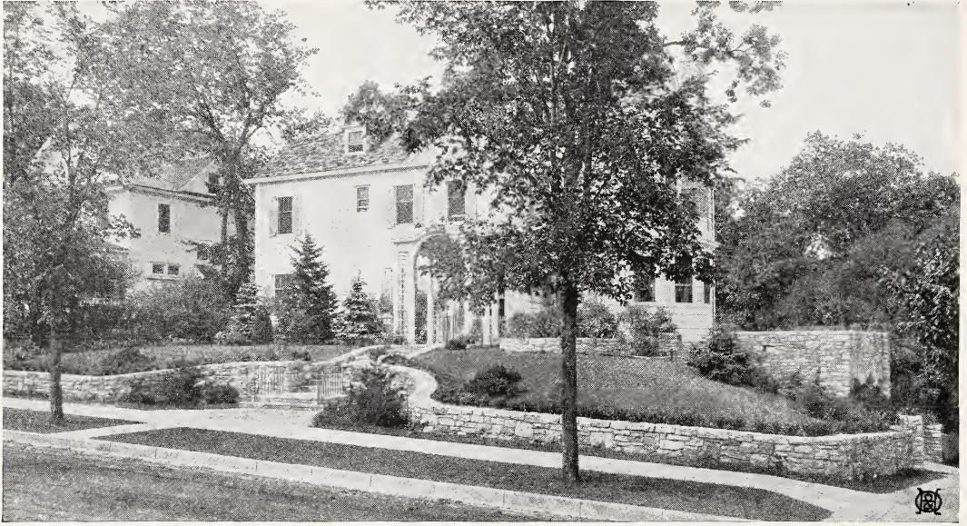
The all-year-round beauty of the Evergreens is especially enjoyed when they are planted near the house. Photograph taken sixty days after the lot was graded and planted. Home of Mr. Louis L. Swarthe, Minneapolis
