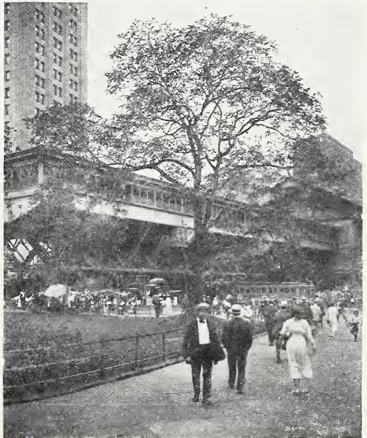
At the end of Brooklyn Bridge, right in the heart of busiest New York, this Tree of Heaven from our Nurseries is growing vigorously, demonstrating its worth for planting under congested city conditions.
