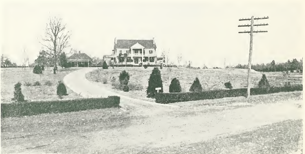
Taken just as planting was commenced.
