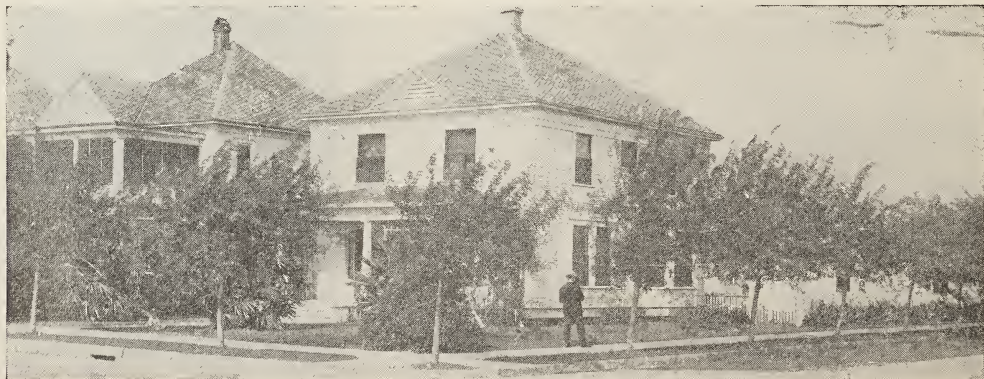
Planting of Griffings Arizona Ash, Second Year
