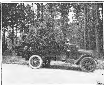
Concrete Road to the Nursery Through the Pines.
