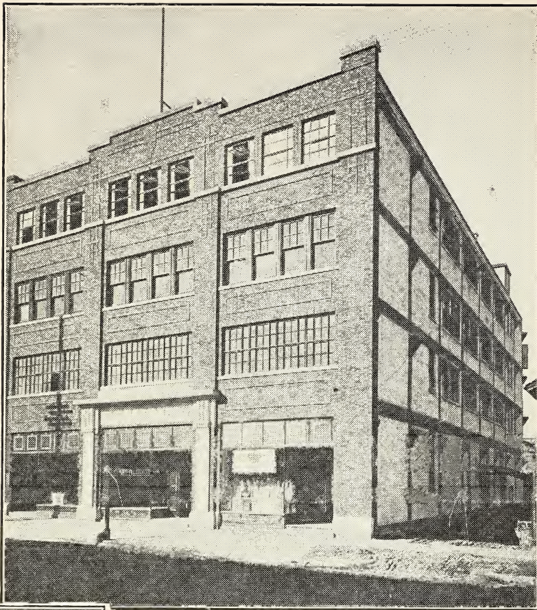
Olds Building, 720, 722 and 724 Williamson St., Madison. Built of Steel, Brick and Concrete and Strictly Fireproof. The Structure is 60 by 125 Feet, Four Stories and Basement.
