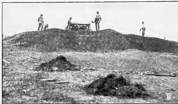
An unusual construction scene in New York City: building traps on the new "Subway" Golf Course, situated in Brooklyn, centered amid a two and a half million population.
