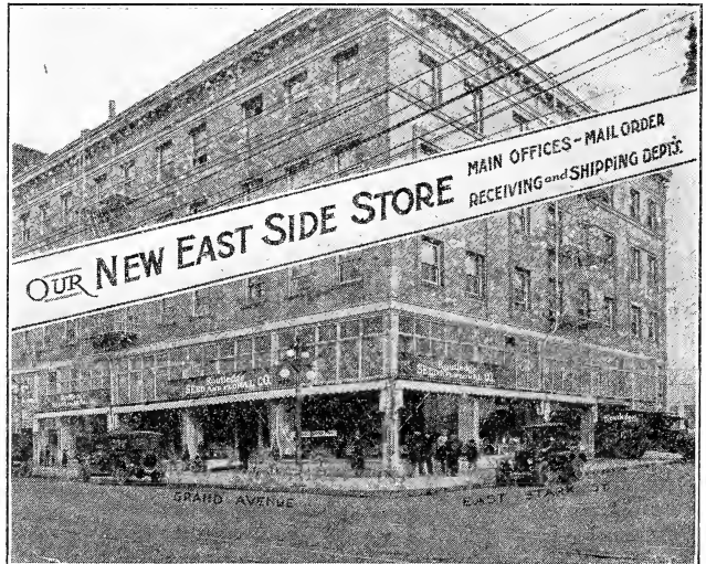
STORE, WAREHOUSE AND MAIN OFFICE, CORNER GRAND AVENUE AND EAST STARK STS.
