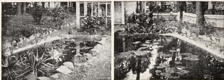
The finished pool, built by Mr. R. E. Bishop, according to specifications here given
