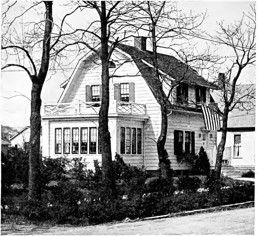
School Practice House planned and demonstrated by students of the civics classes, Washington Junior High School, Port Huron, Mich., 1925. The school boys and girls had charge of the Better Homes Campaign in Port Huron. The cost of building this house was $4,812.
