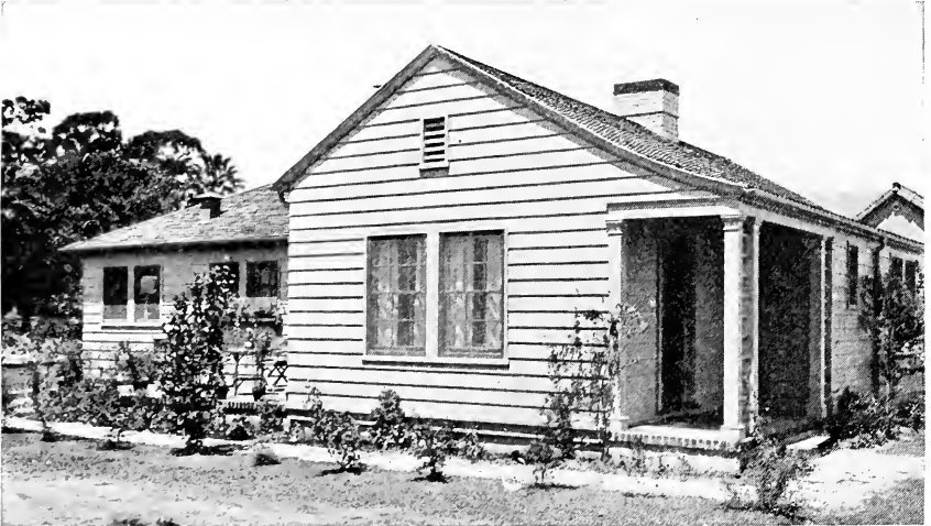
Another view of Demonstration House No. 1 at Santa Barbara, Calif. Note the irregular flags in the walk, the planting, and the open porch at the rear
