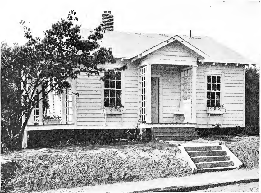
Exterior of Demonstration House No. 3, Atlanta, Georgia, 1925. This house, which contains four rooms, was furnished and demonstrated by a subcommittee of negroes, as a Better Home for people of their race. The cost of construction was $2,150. The lot upon which it stands is valued at $850. Erected from plan No. 4-A-8 of the Architects' Small House Service Bureau.
