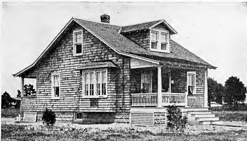
Six-room Demonstration House at Rehoboth Beach, Del., 1925. This house, completely finished throughout, and with a full concrete basement (but no furnace) cost $2,650
