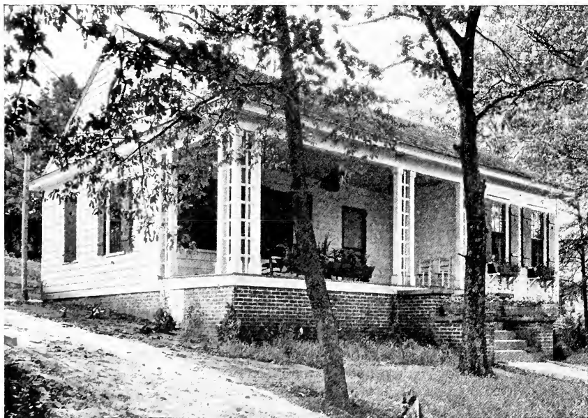
Attractive six-room house demonstrated by Better Homes Committee at Greenville, S. C. 1925. The advantage of good natural surroundings is well illustrated in this photograph. Note also how the architect has allowed for the slope of the ground. This house is stated to have cost $3,500 to build.
