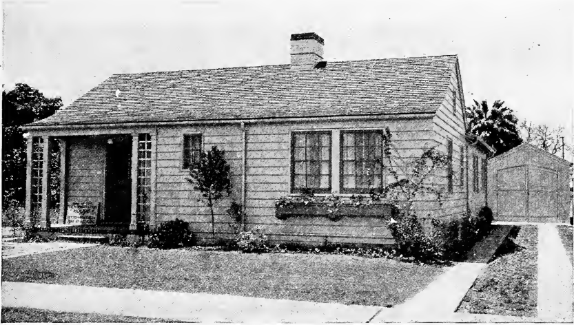
The six-room Demonstration House No. 1 at Santa Barbara, Calif., 1925. This house cost $6,109 to build. The planting around the house adds a great deal to its appearance
