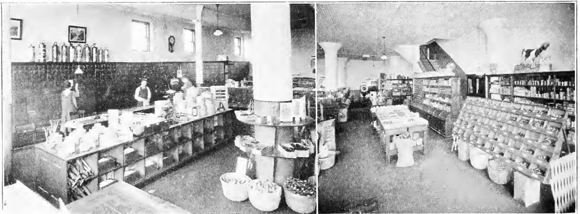
Interior view of Gould's large retail store.
