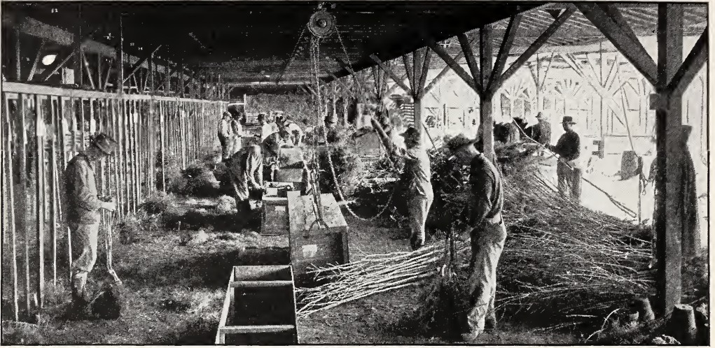
Interior of our packing-house at Glen Saint Mary
