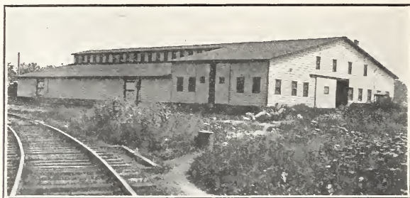
Packing house and storage cellar, Princeton Nurseries. They are on our own siding which insures the minimum of exposure when loading and facilitates rapid shipment. We specialize in carload orders for which no charge is made for packing.
