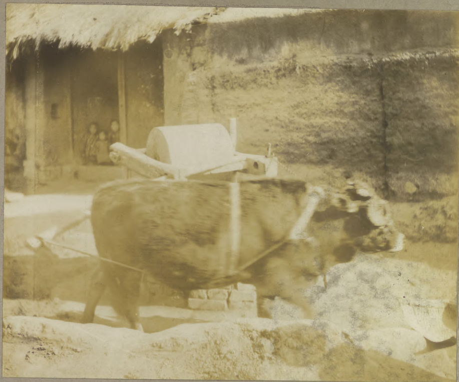
No. 12001. "A blind-folded ox, used as motive power in drawing the stone roller that hulls and grinds all sorts of grains."
