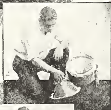
3—Press Setter 1/4-inch in ground.
