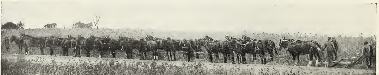
Digging Trees on Green's Nursery. Plenty of Horse Power Enables Us to Keep the Blades of the Tree Digger Down Deep. This Insures an Abundance of Fibrous Roots.
