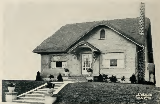
BUILDING DONE—RESIDENCE EAST 14TH N. AT STANTON
