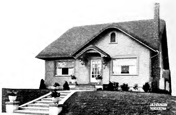
BUILDING DONE—RESIDENCE EAST 14TH N. AT STANTON
