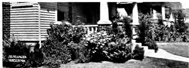
FOUNDATION PLANTING EAST 16TH N. NEAR SHAVER Irish Juniper, Port Orford Cedar at front entrance. English Laurel in corner with Hydrangea, Laurustinus, Evergreen Bush Honeysuckle and Golden Privet
