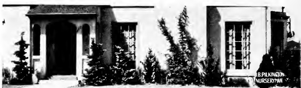
BASE PLANTING STUCCO HOUSE, E. 30TH N. AT THOMPSON Japan Cypresses at entrance, Firethorn at chimney, Cypress at corner
