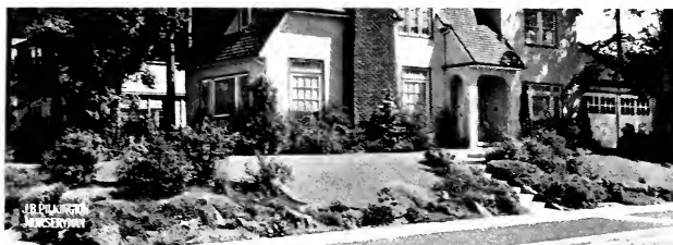
AN IRVINGTON RESIDENCE, THOMPSON ST. AT EAST 32ND Note the plant bordered entrance steps, Veronica, Abelia and Cotoneaster. Pyramidal Japanese Cypress against chimney and Lawson Cypress at corner of house. Planting limited to foundations and borders, leaving open lawn
