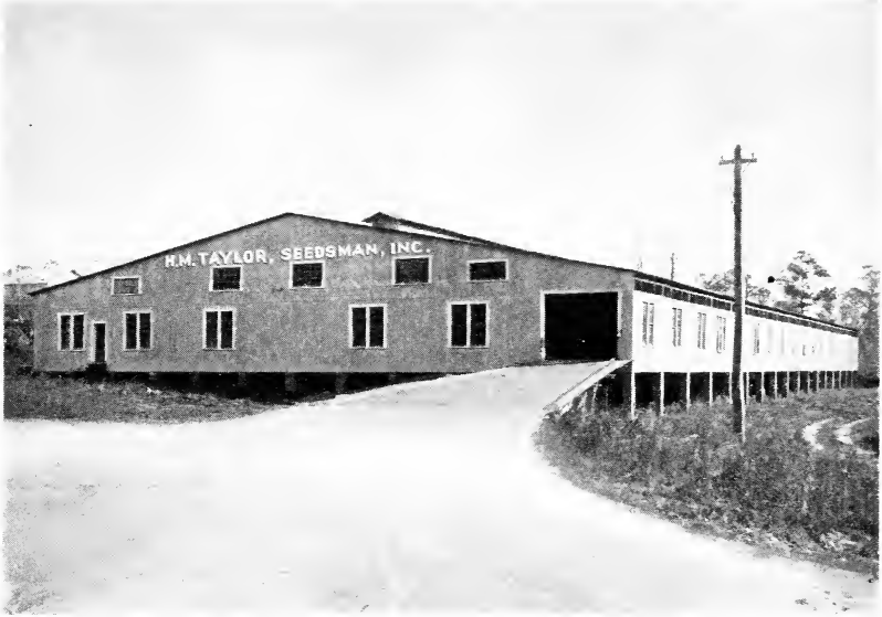
Our Quincy Warehouse Contains 43000 Square Feet of Floor Space.
