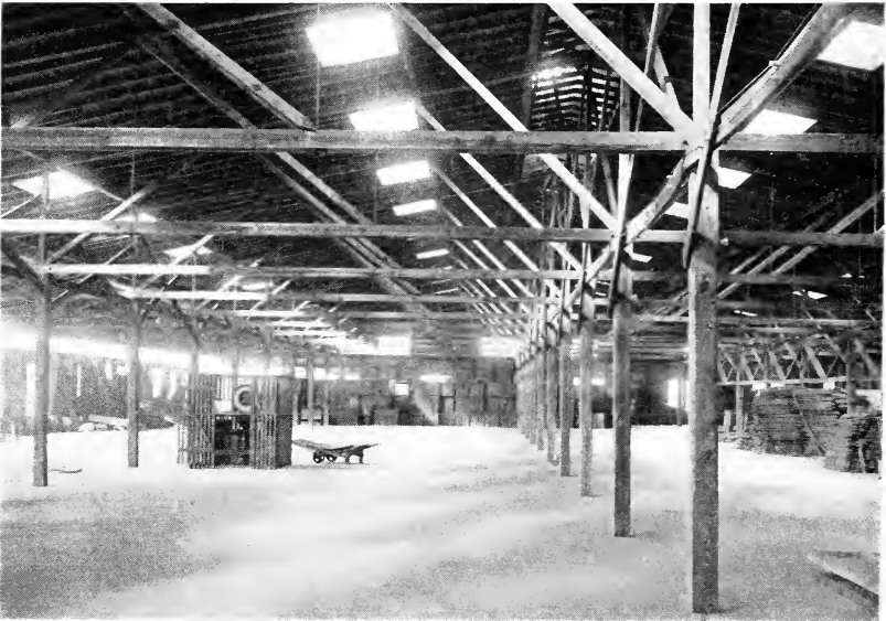
Partial View of Interior of our Quincy Warehouse, Nearing Completion Note Exceptional Ventilation and Equipment
