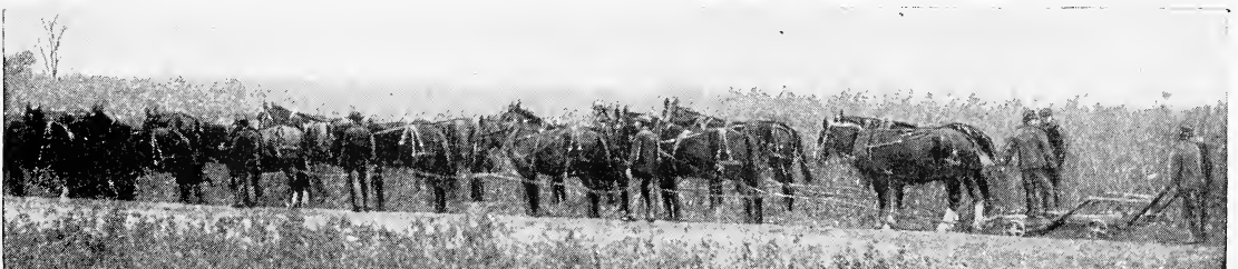
Digging Trees in Green's Nursery. Plenty of Horse Power Enables Us to Keep the Blades of the Tree Digger Down Deep. This Insures an Abundance of Fibrous Roots. Twenty Horses are Used.
