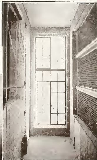
Directly below is shown the automatic oil heating plant; also the mammoth fan and piping. At the extreme right the air intake and steam-heated radiators which heat the air drawn in by the fan.
