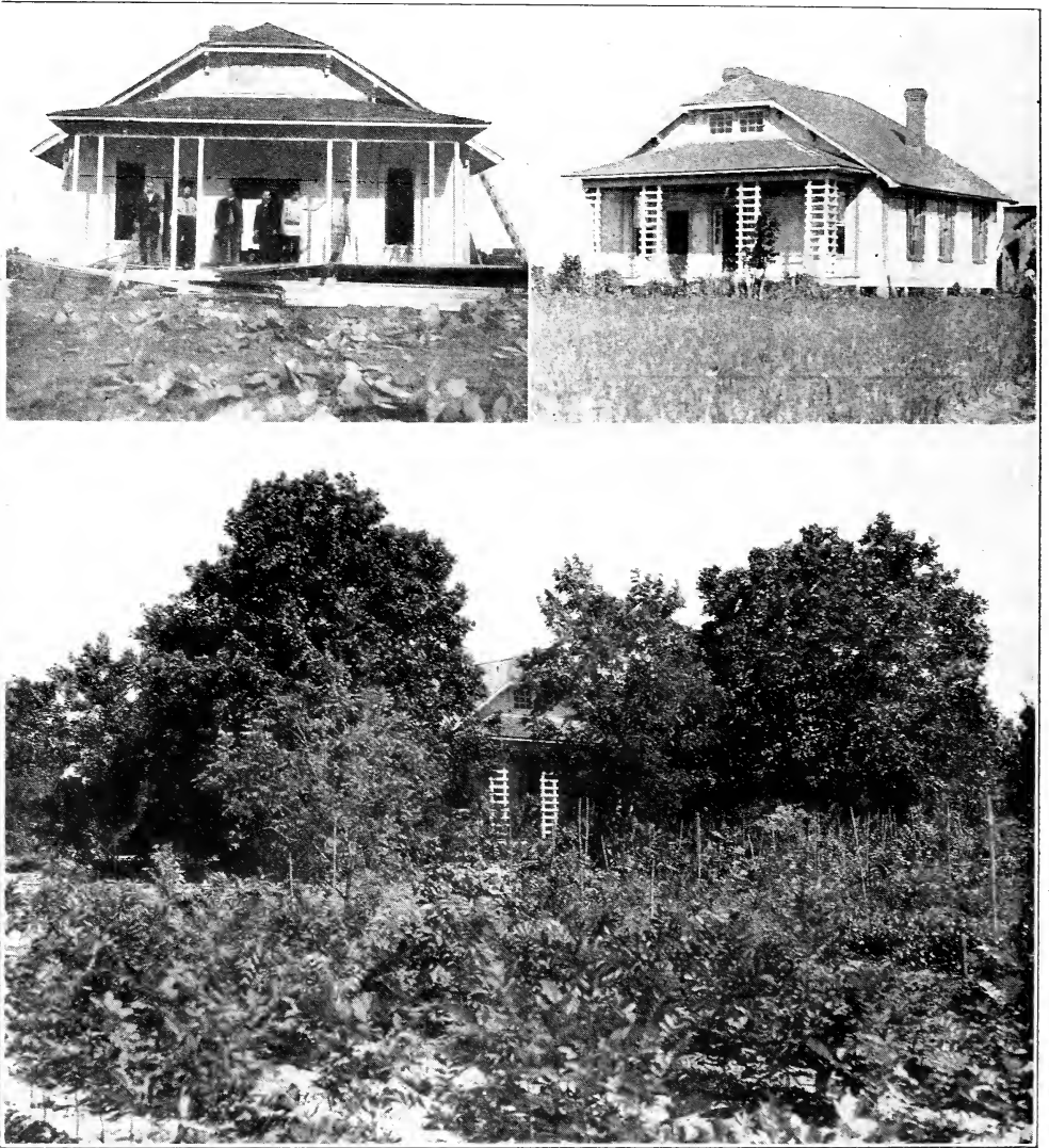
Upper Left:—Building house in 1914.
