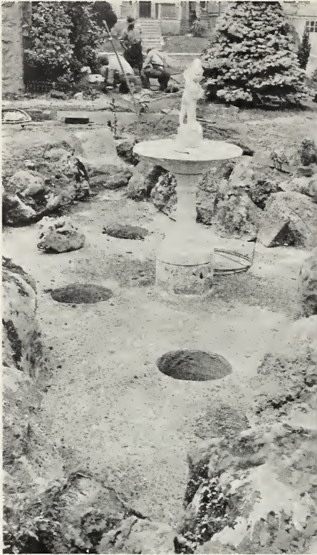
Construction Details of Lily Pool Before Completion
