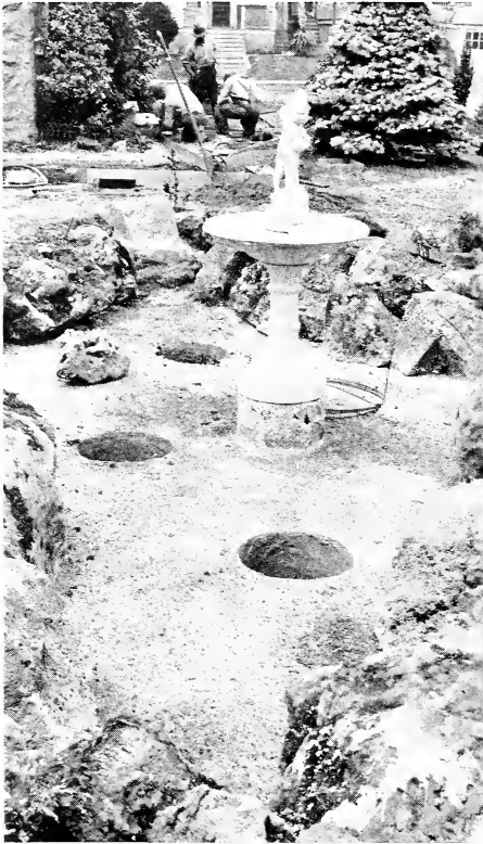
Construction Details of Lily Pool Before Completion
