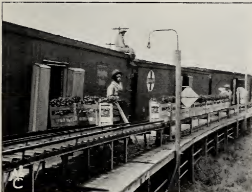
Above is one of the loading stations of the American Fruit Growers, Inc., Sanford, Fla., and the loading of a solid train of our No. 14 Golden Celery.
