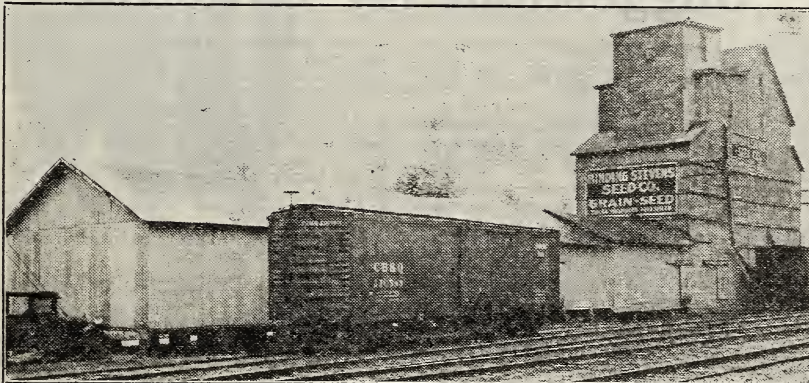
Tulsa Mill and Warehouse on the Midland Valley Tracks
