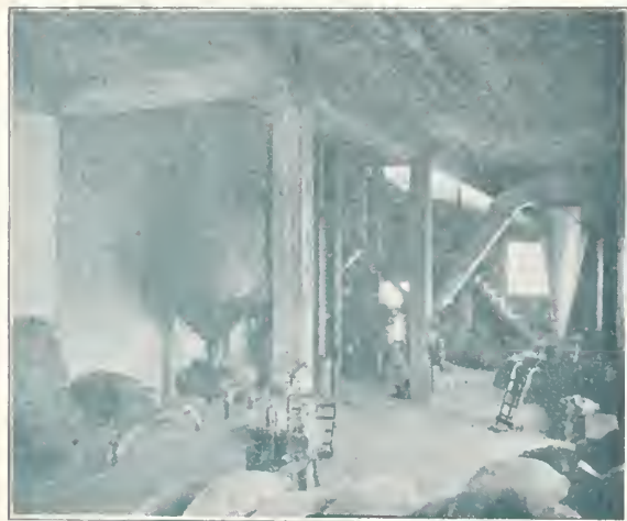
View of Seed-Cleaning Equipment
