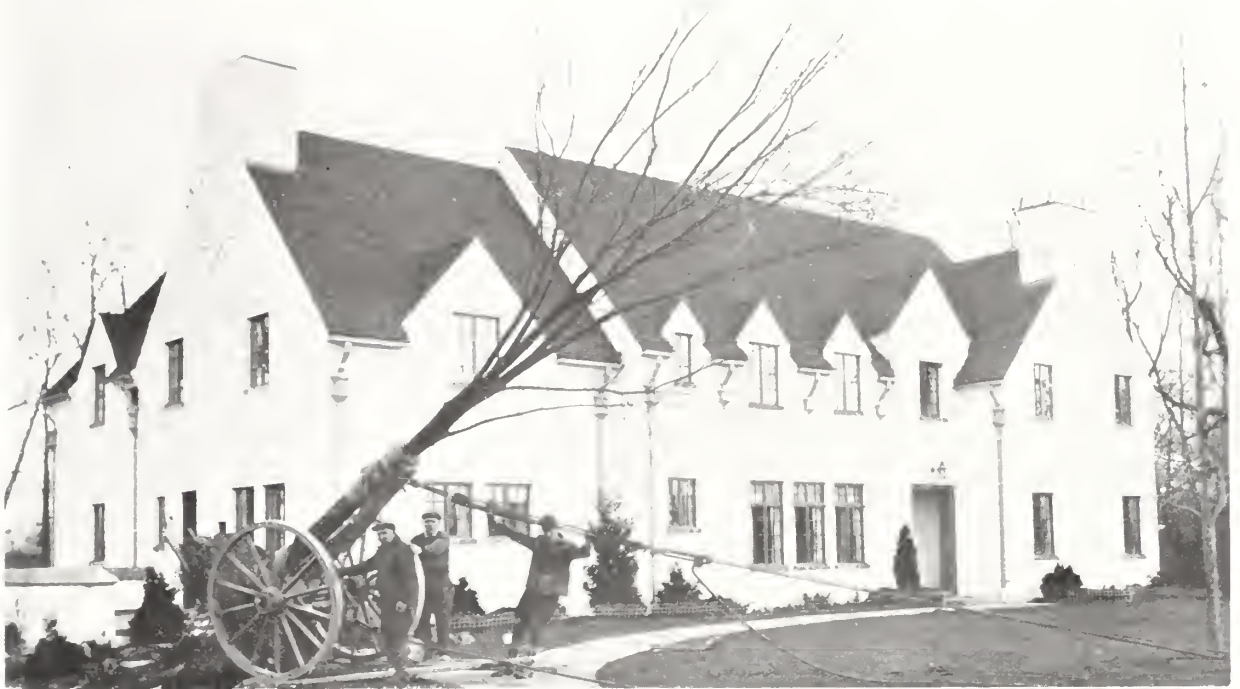
New residence of Adolph Stuber, Esq., Ambassador Drive, Rochester, N. Y. Grading and Seeding—Plans and Planting—Plants and Trees—Wall and Step Construction—photo shows our tree moving crew planting a 12 inch Elm selected at Glenwood Nursery. Entire job by Glen Brothers, Inc., Landscape Dept.
