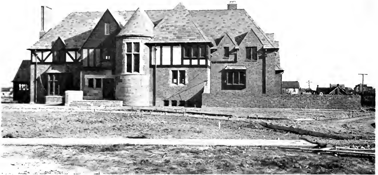
Residence of A. B. Shultz, Esq. Amherst Estates, Buffalo, N. Y. Photo taken Winter 1931. See photo below for planting results in three months.
