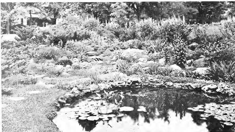
This pool is constructed so that no concrete shows. Porous rocks over-hang the edge of the water so that the water covers half of the rocks. This gives a moss covered edge and more of a natural and pleasing appearance
