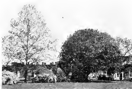
Front view of our plant at Neosho.
