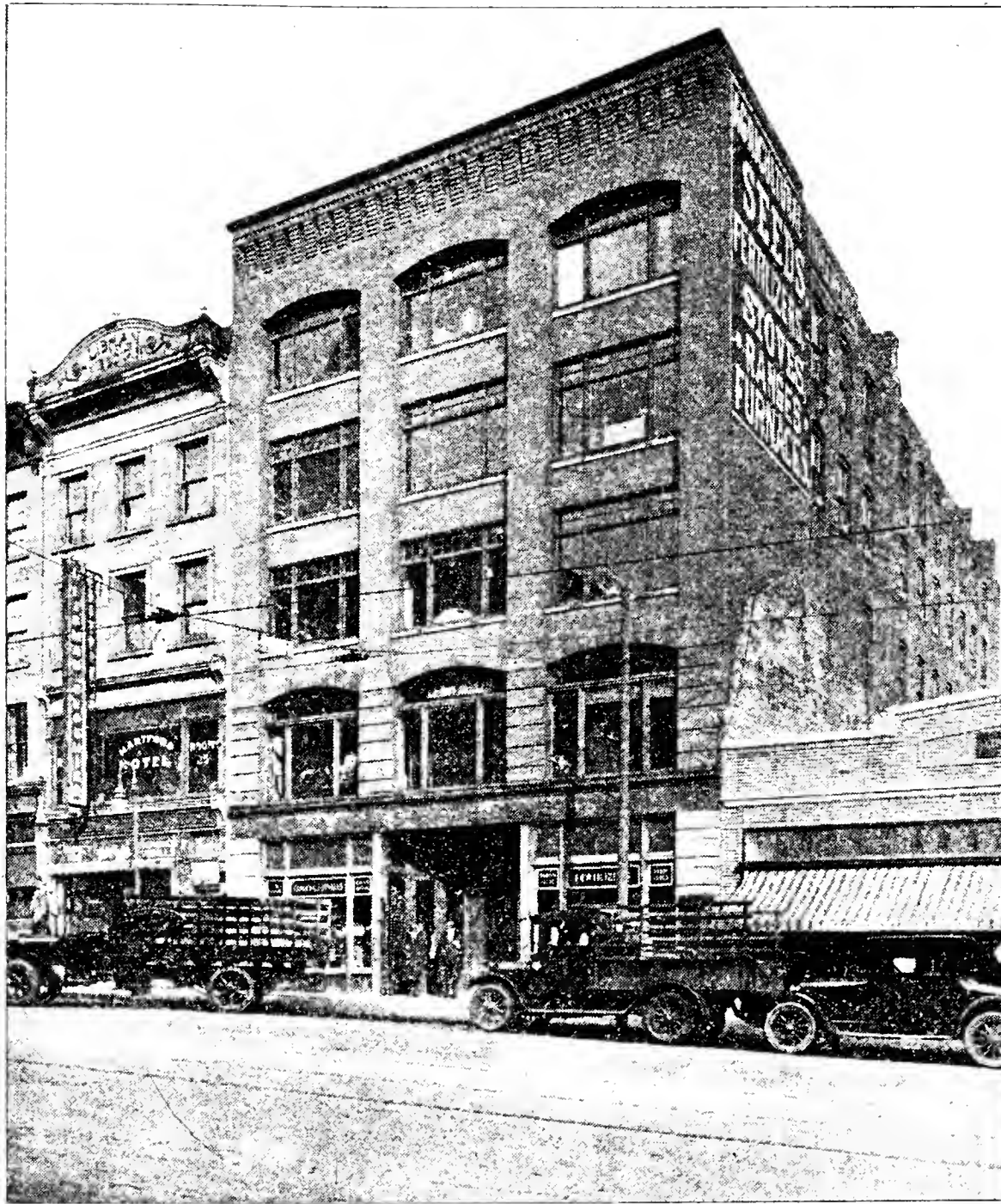
Offices and Agricultural Warerooms at 168 State Street, Hartford, Conn.
