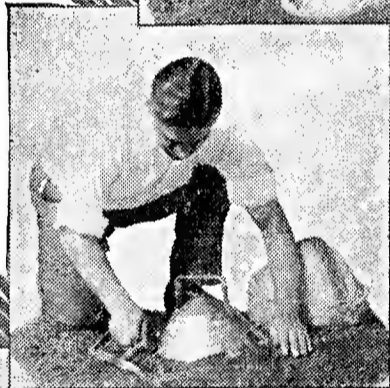
Tamp soil around edge of SETTER
