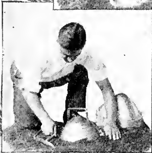
Tamp soil around edge of SETTER
