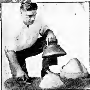
Tamp soil around edge of SETTER
