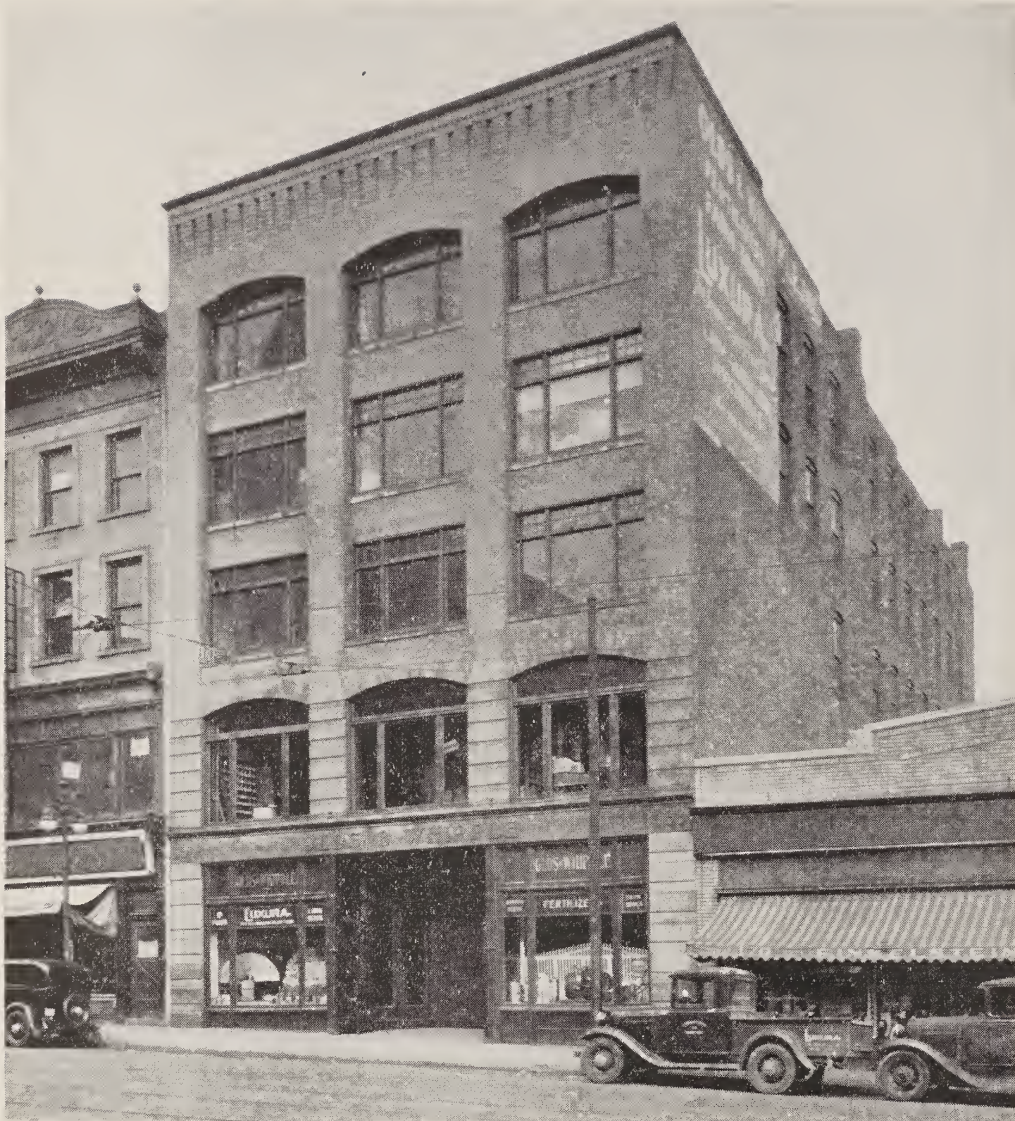
Offices and Agricultural Warerooms at 168 State Street, Hartford, Conn.
