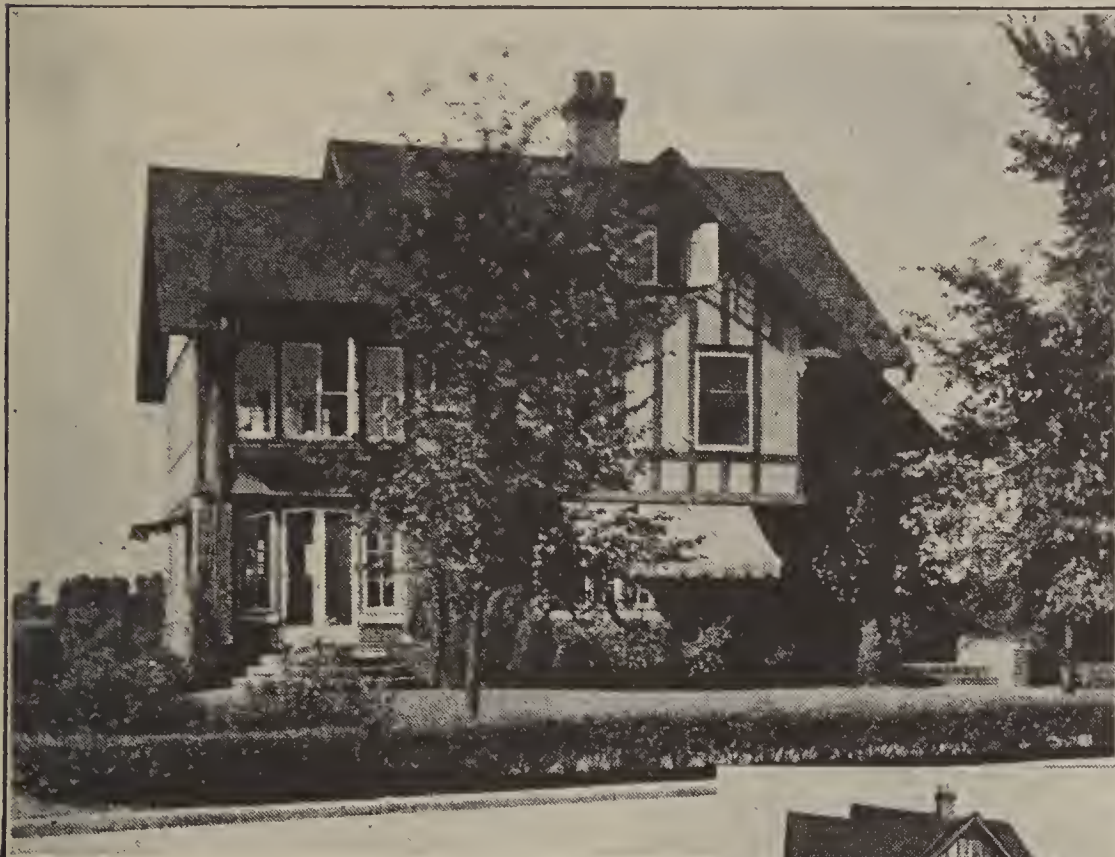
Through the Use of Proper Materials Immediate Results Are Possible
